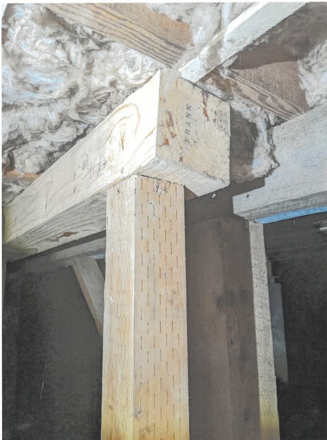
FIGURE 17: ONE OF TWO LOCATIONS WHERE POSTS AND BEAMS WERE INSTALLED TO COMBAT MOISTURE DAMAGED ELEMENTS AT EAST END OF STRUCTURE. IT IS UNKNOWN WHEN THESE WAS INSTALLED.
