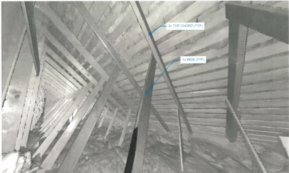
FIGURE 24: FRAMING OF MAIN HALL ROOF, CONSISTING OF WOODEN TRUSSES WITH 2X CHORDS AND 1X WEBS.
