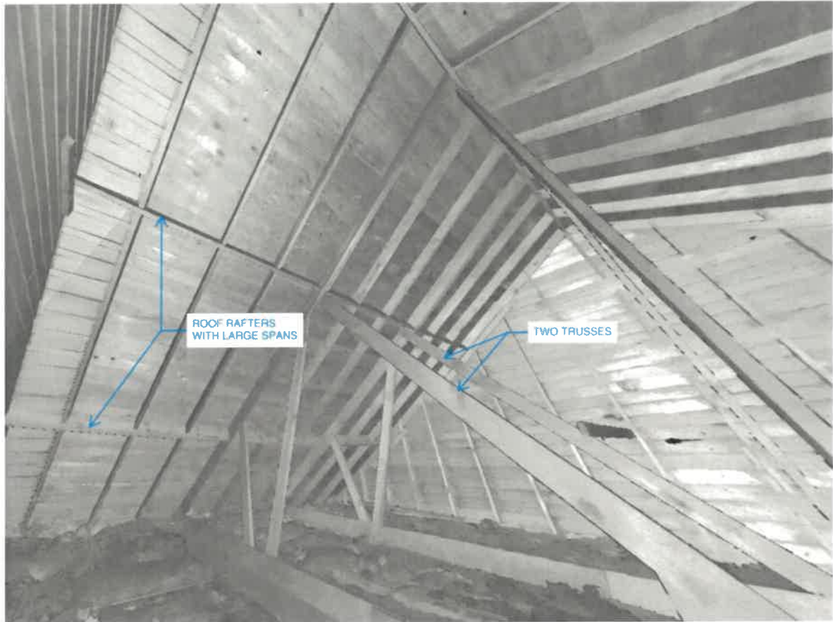
FIGURE 25: ROOF FRAMING AT COSTUME ROOM ADDITION, CONSISTING OF 2X ROOF RAFTERS WITH TWO TRUSSES.
